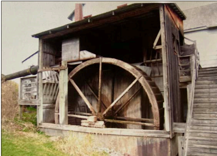
AN 18 FOOT-SIX INCH waterwheel with a three foot face powered the Kister mill. A new one will be installed, hopefully this year.
